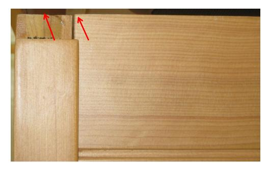
Note: When wall panels are connected in place properly the corners will be level and flush on top.
