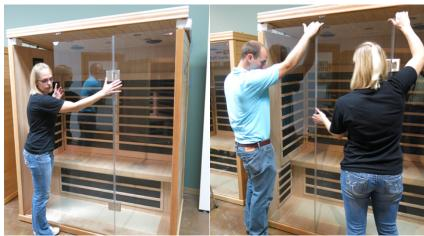
**Note:** Secure the door from falling open and breaking while setting the Front Wall panel. It may be helpful to use your knee to help push in the Front Wall panel while lowering into place.
