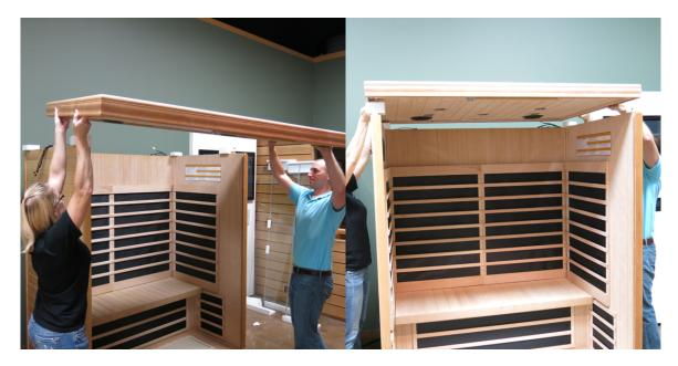
• Once the Ceiling panel is lined up directly above the Wall panels; insert the wires harnesses from the wall panels into the holes in the Ceiling panel.
