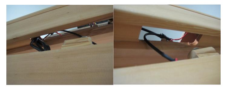
Note: Position the cam locks on the top of the Left & Right Wall panels as shown above.
